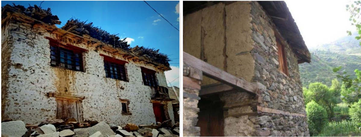
Figure 87 Dry stone construction & Mud construction
