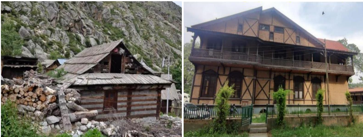
Figure 86 Kath-Kuni construction & Dhajji –Diwari construction
